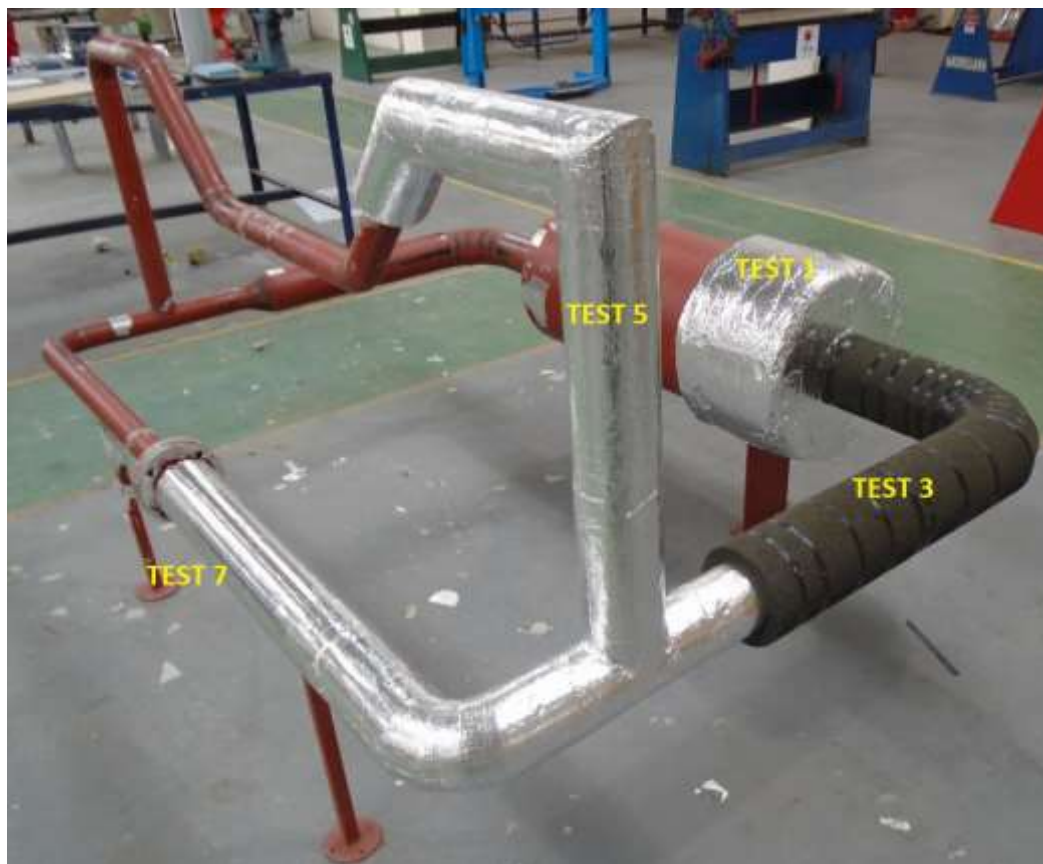
Photograph of completed tests 1-8
